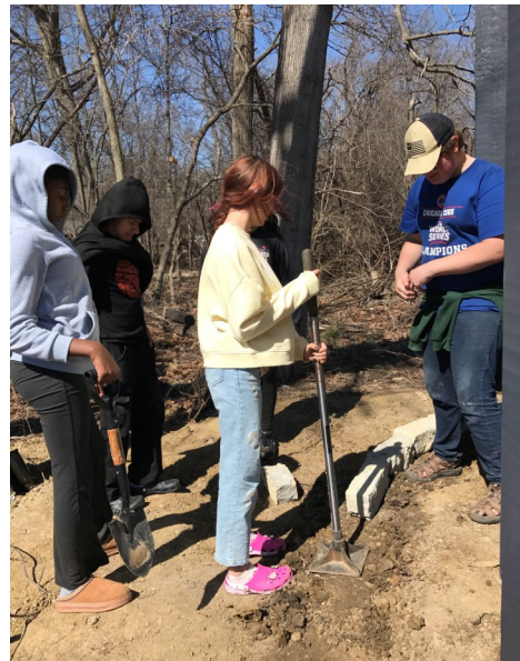
Falcons Anna, Serenity, Ben and Aaron work to level the foundation for the stone wall.
